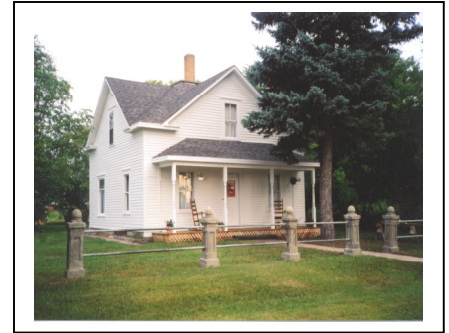
The restoration of the exterior of the Melby-Rogness Home was nearly completed at the time of Manfred Days, July 14-15, 2001.
